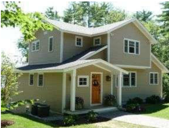
Road side of house
